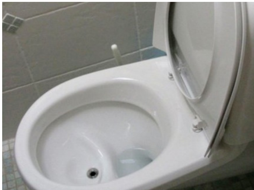
Separating urine from the wastewater of residences or public facilities through the use of urine-diverting toilets or urinals can potentially reduce phosphorus loading to onsite wastewater systems by as much as 50 percent.
