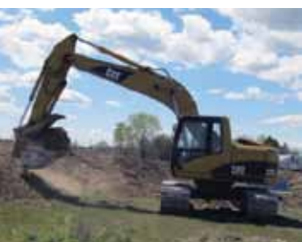
PARKER HORN DREDGING PREPARATION
