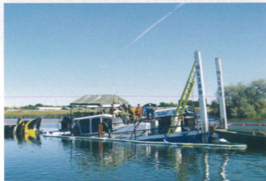
Dredge site with spill containment boom in place.
