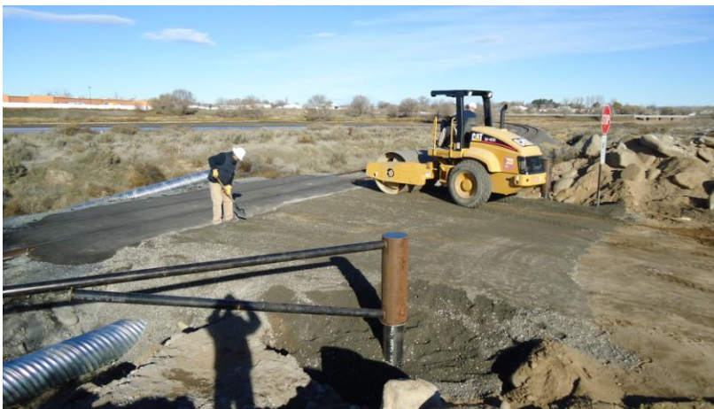
Planning Pays Off – Pre-dredging Projects Underway
