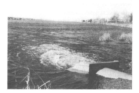
Discharge of Dilution Water Pumped into Pelican Horn summer with dilution water available since 1985. The pump discharge rate was constant at about 50 cfs. Typically, water is transferred from Parker Horn to Pelican Horn throughout the spring-summer period. Pumping usually starts in April after dilution water has improved Parker Horn guality in the vicinity of the pump intake structure.
